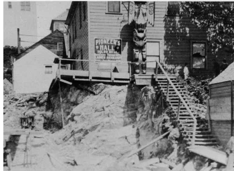
1925 late View from Front Street. Note totem pole, POA sign and clapboard siding on SW (Front Street side). Note covered entrance on NW (Pioneer Alley) side. (Excavation on the left is for the Citizens Light and Power building)
