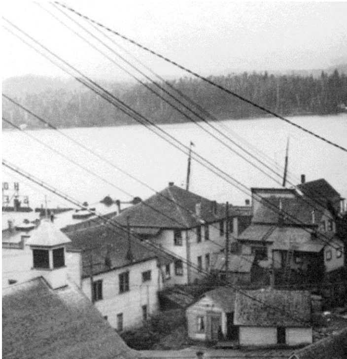
1913 circa N corner of building. Note flagpole still present, roofline symmetric, and no doors onto Pioneer Alley.
