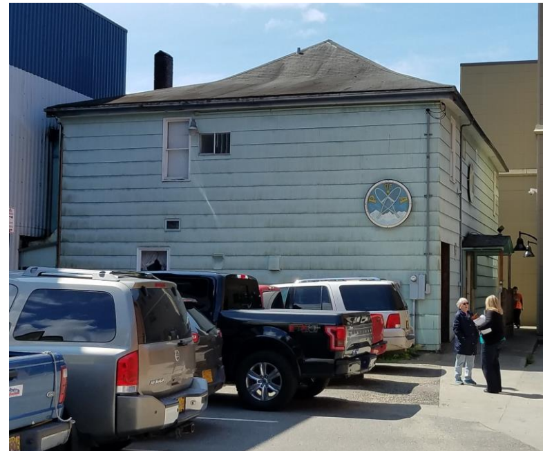
2019 NE (Parking Lot) side of building.
