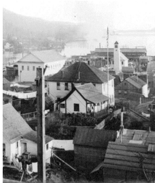
1904 NW (Pioneer Alley) and SW (Front Street) side of building.
